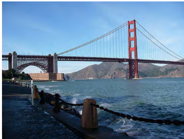
Figure 4.20 Unless an infinite tension is exerted, any flexible connector—such as the chain at the bottom of the picture—will sag under its own weight, giving a characteristic curve when the weight is evenly distributed along the length. Suspension bridges—such as the Golden Gate Bridge shown in this image—are essentially very heavy flexible connectors. The weight of the bridge is evenly distributed along the length of flexible connectors, usually cables, which take on the characteristic shape. (credit: Leaflet, Wikimedia Commons)
