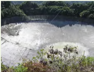
Figure 27.28 A 305-m-diameter natural bowl at Arecibo in Puerto Rico is lined with reflective material, making it into a radio telescope. It is the largest curved focusing dish in the world. Although D for Arecibo is much larger than for the Hubble Telescope, it detects much longer wavelength radiation and its diffraction limit is significantly poorer than Hubble's. Arecibo is still very useful, because important information is carried by radio waves that is not carried by visible light. (credit: Tatyana Temirbulatova, Flickr)
