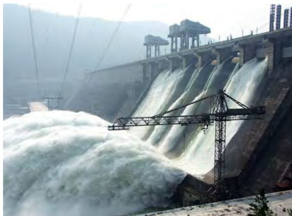
Figure 7.38 Hydroelectric facility (credit: Denis Belevich, Wikimedia Commons)
